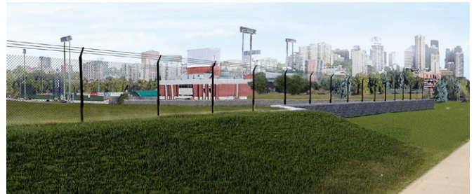
This rendering shows how the flood barrier might look once complete. The barrier will use a combination of grass-covered embankment and concrete wall.
