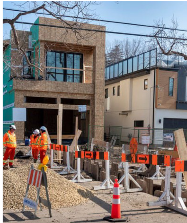
Residential new service connection under construction
