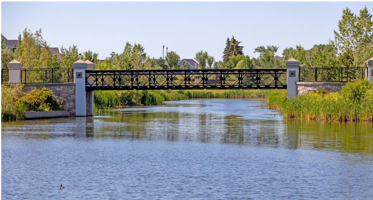
The Griesbach Stormwater Management Facility
