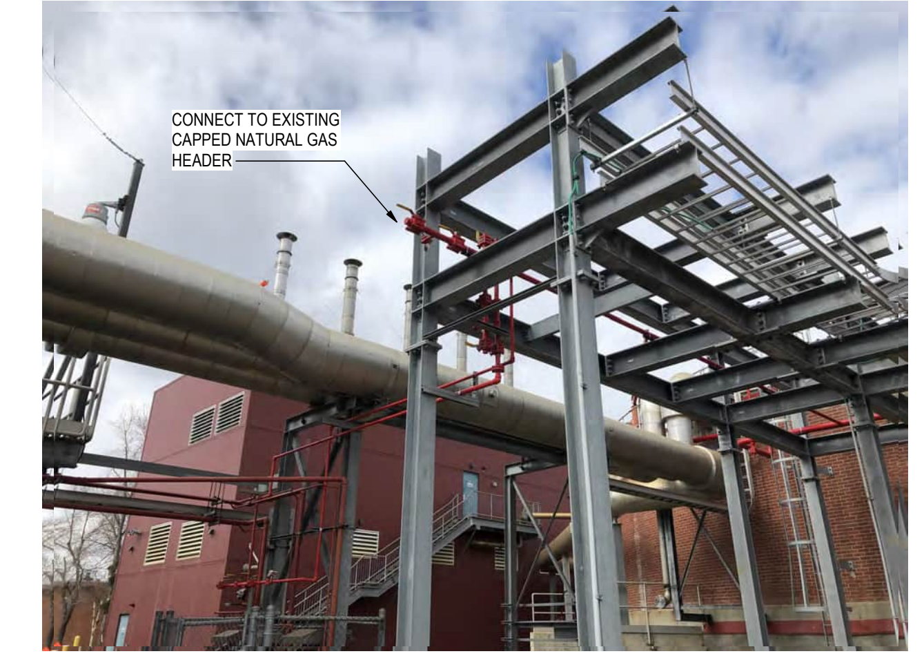
2 SITE PHOTO - NATURAL GAS TIE POINT N.T.S.
