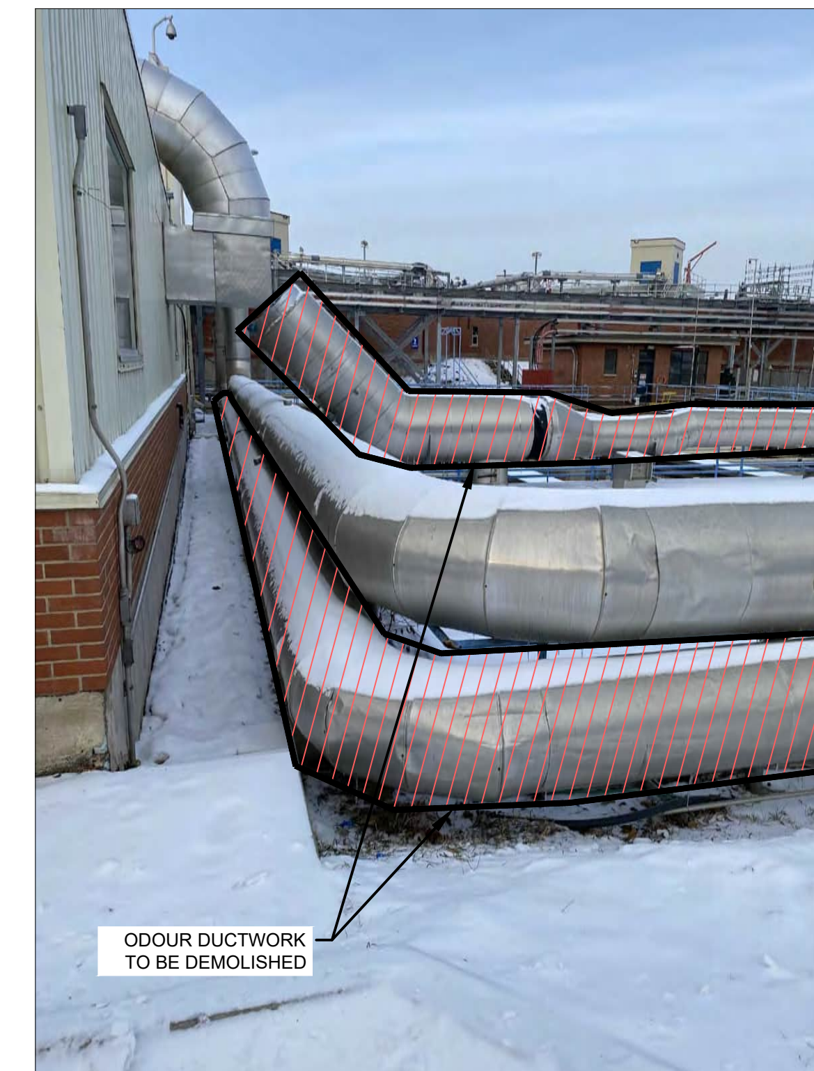
3 PHOTO 3 - LOOKING NORTH NTS
