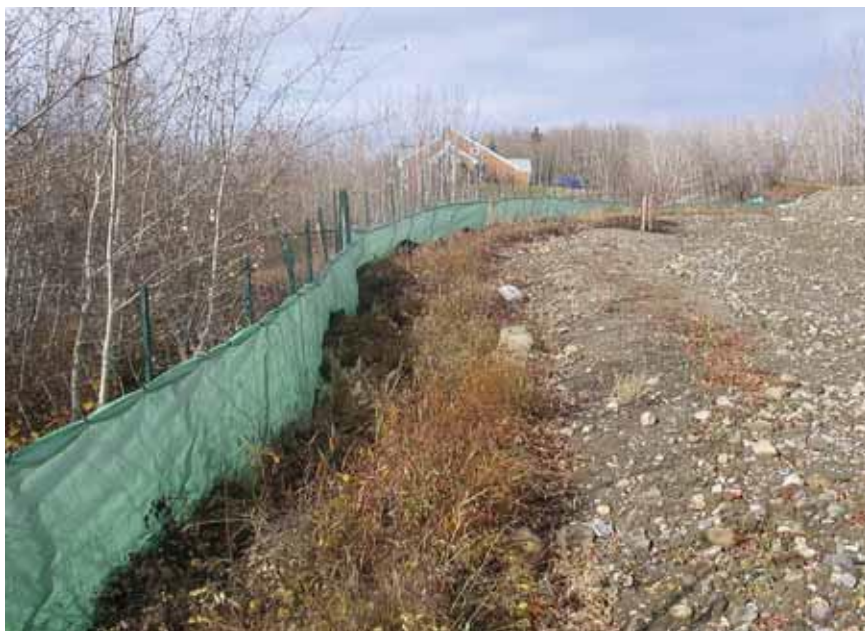
21 Vegetated buffer used as a Transport Control BMP
