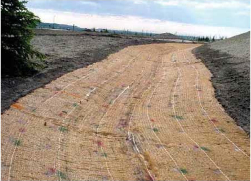
20. Erosion Control Blanket In a future grassed waterway
