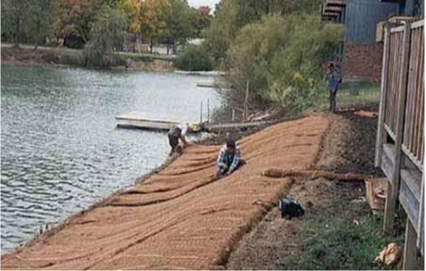
17. Rolled Erosion Control Protection (RECP) being installed along a river bank
