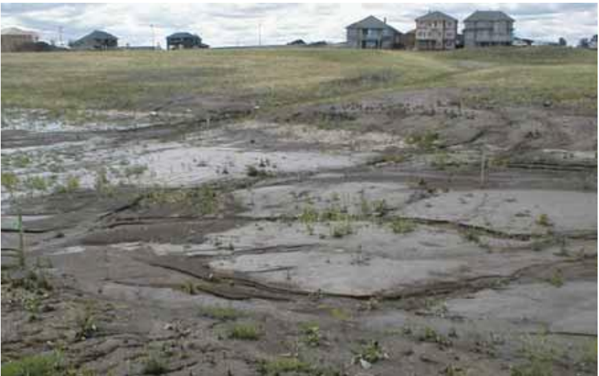
1. Stripped and graded site results in no protection of soils, formation of gullies, and concentrated stream flow
