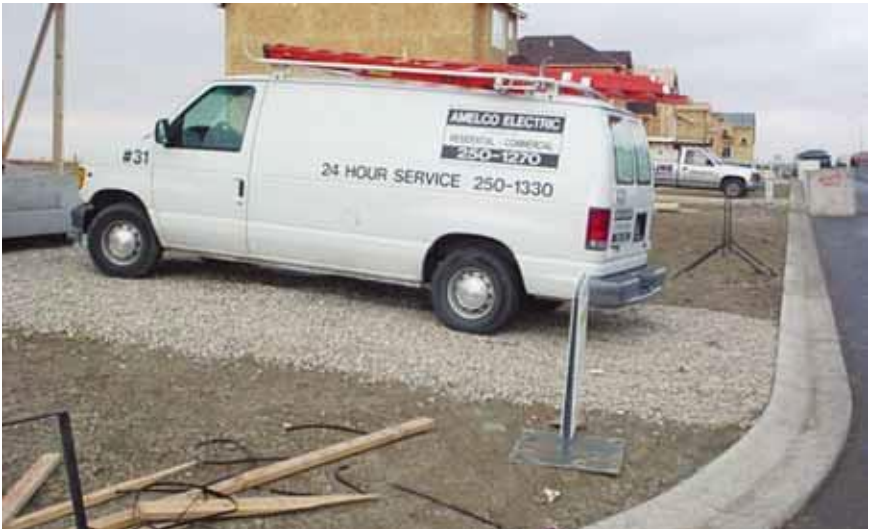
44. Gravel pad reduces off-site mud-tracking
