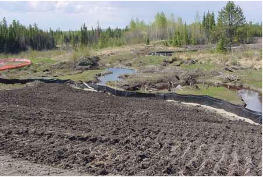
24. Silt fence used as perimeter fence
