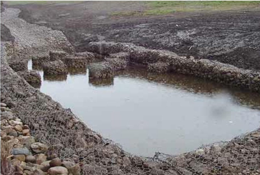
36. Gablon energy dissipation structure
