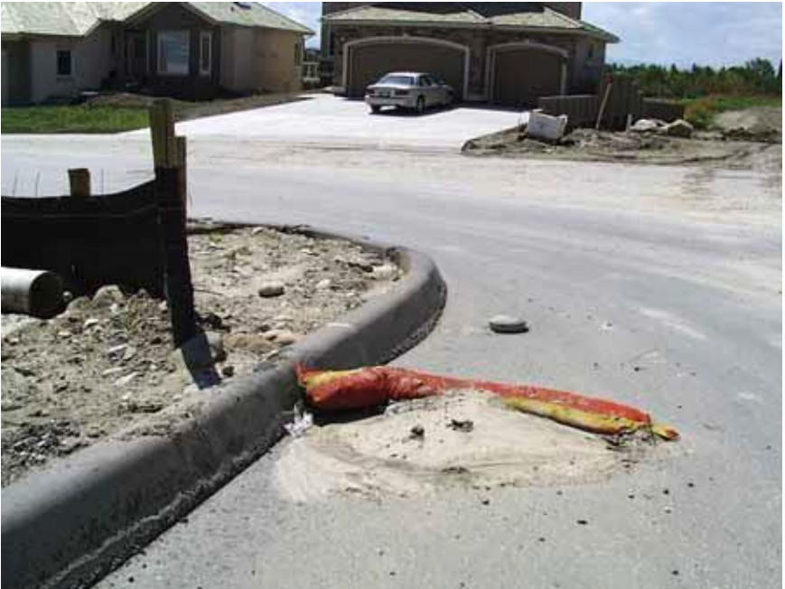
42. Rock sock used for Inlet protection
