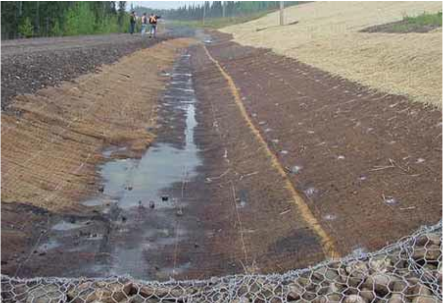
18. Channel protection using RECP
