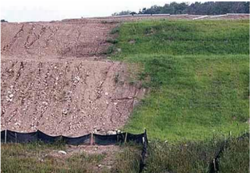
13. Rills forming along stripped slope; vegetated slope resists erosion. Terracing also breaks up slope and, where properly constructed, helps resist erosion.
