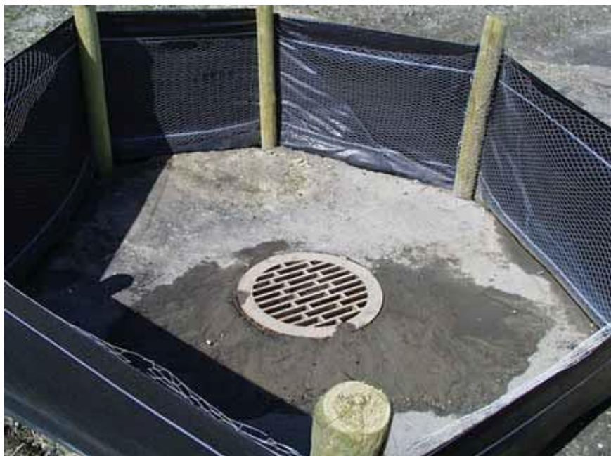
40. Good installation, but is the fence trenched
