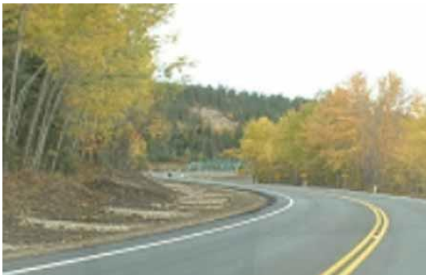
27. Rock ditch checks along highway
