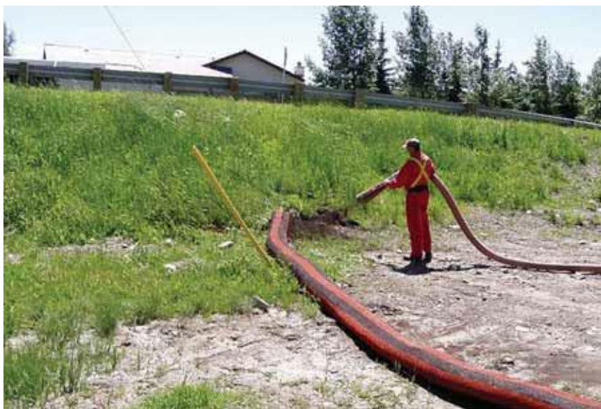
32. Seeding around a sediment trap sock filled with compost
