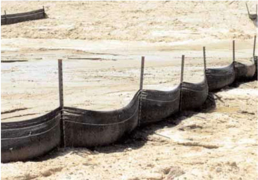
26. Well installed silt fence, but requires maintenance to remove sediment
