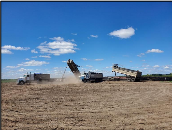
Photograph 3: Biosolids are delivered to the stockpile in NE32. (May 2022)
