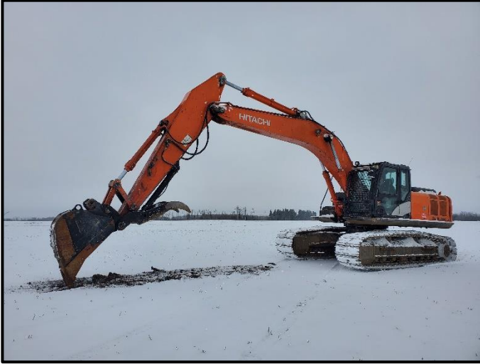
Photograph 1: Excavator digging soil pit for pre-application site assessments. (March 2022)
