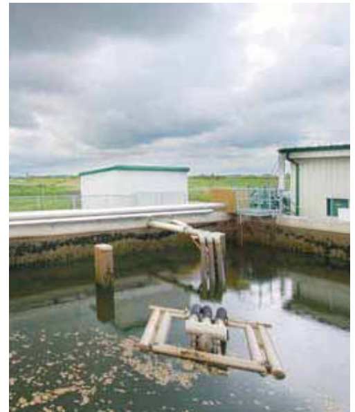
Strathmore WWTP SBR Plant during decommissioning
