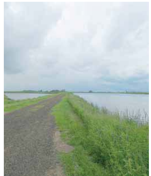
Strathmore WWTP Storage Lagoons
