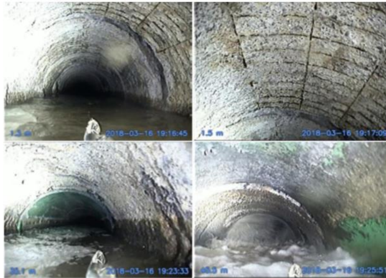
Figure 3.0-1 Deterioration of Small Trunks
